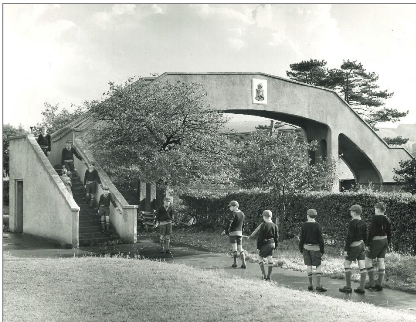
The Junior School Footbridge (1960s)
